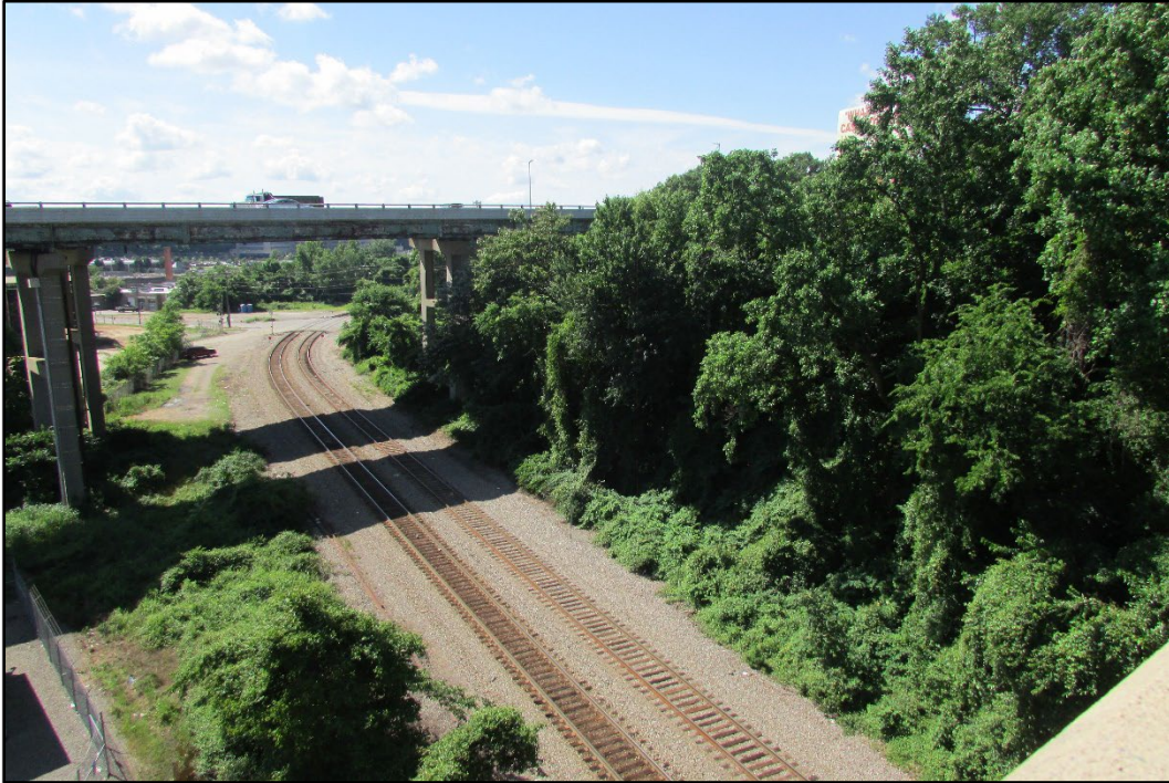
Photo 3: Overview of Rail Corridor in Northeast Corner of Historic Properties, Looking East from North 5 th Street. Existing tracks will be realigned and a third track added.
