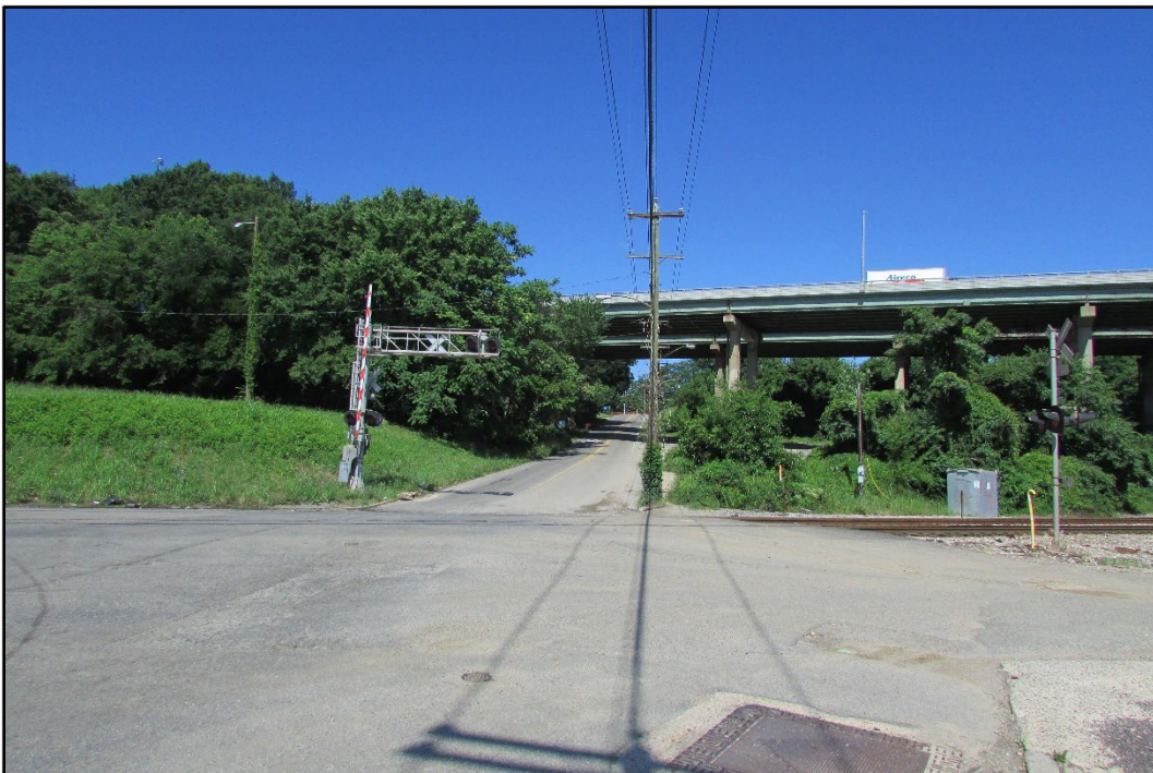
Photo 4: Intersection of Rail Corridor and Hospital Street, Looking West. Hospital Street will be brought over the rail but under Interstate 64 (in background).
