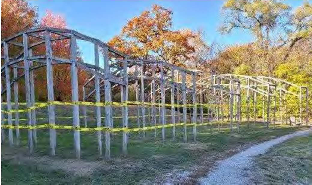
Figure 1. Wood arches north of the pavilion.
