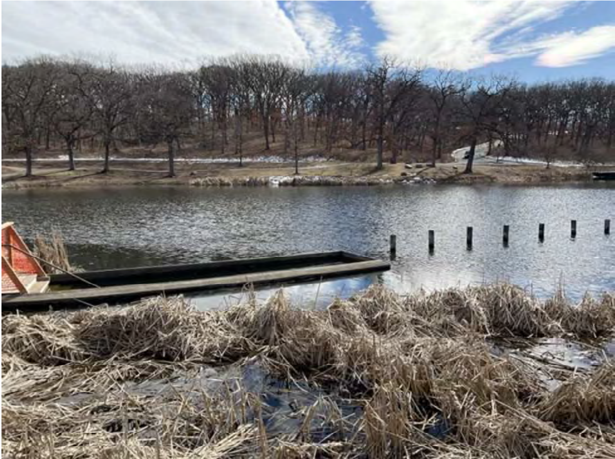
Missing element, inherent decay of post markers in water.
