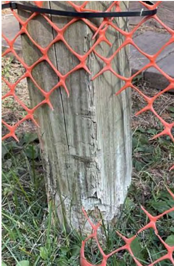
Dry rot (fungal decay) of Pavilion posts
