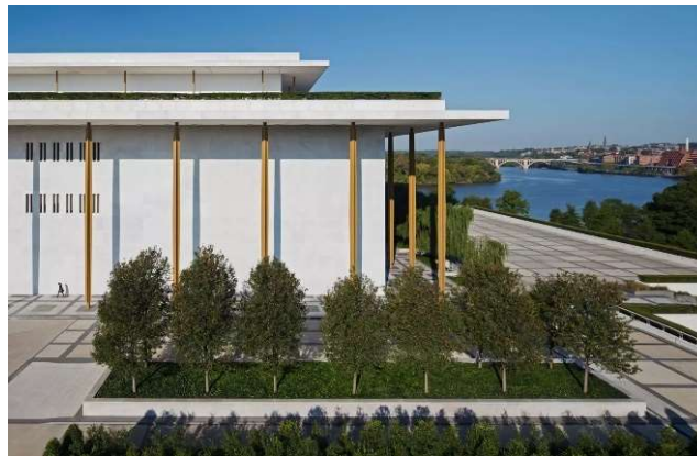
Figure 1. Kennedy Center exterior (prior to fall 2025 alteration of columns, see infra ¶¶ 39-40 & Figure 5). The John F. Kennedy Center for the Performing Arts.
