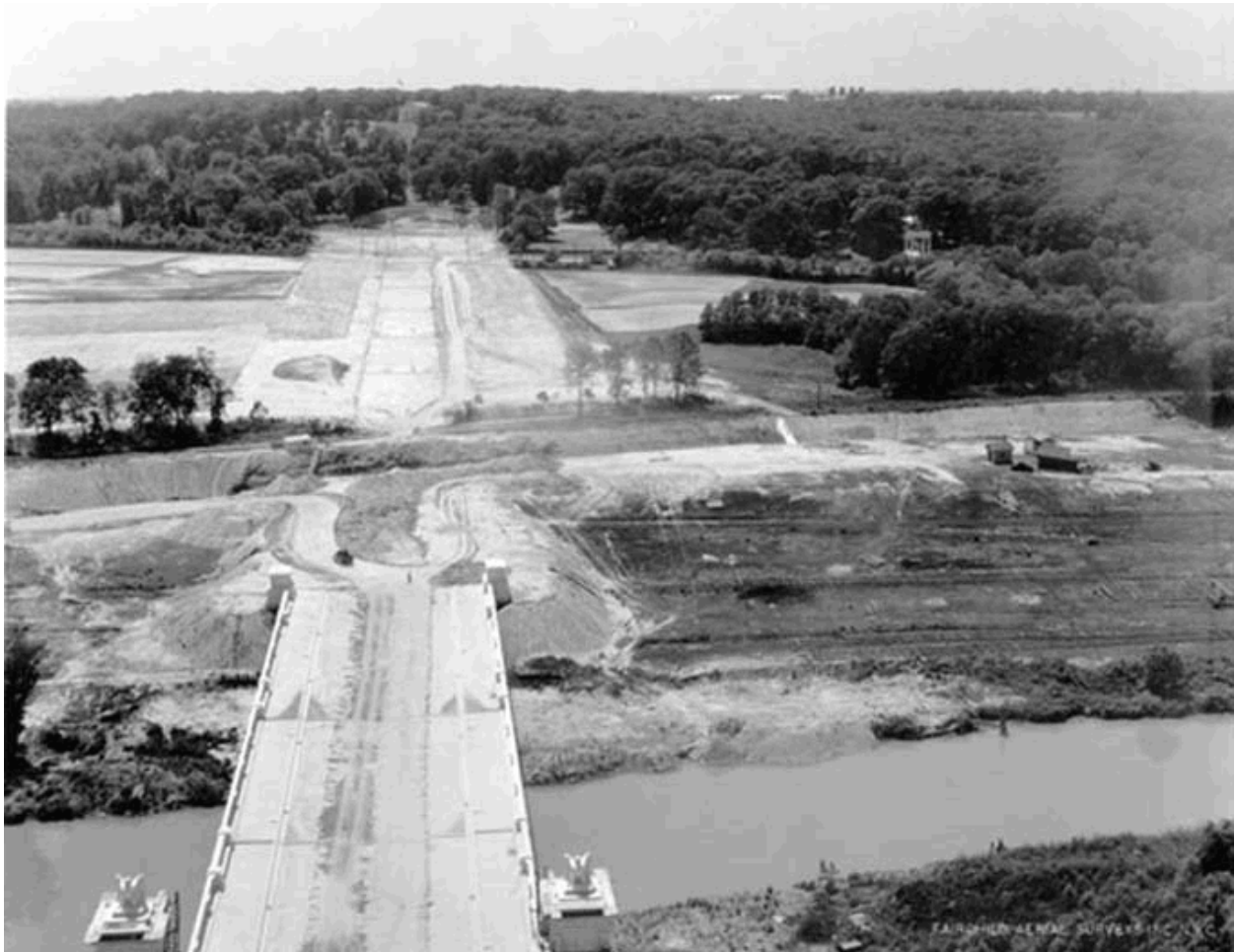
Figure 6 - Cemetery entrance and avenue under construction, June 13, 1931. Boundary Channel Bridge nearly completed. Line of trees in middle range mark former railroad/canal. (NPS/NCR: Fairchild Aerial, 17665)
